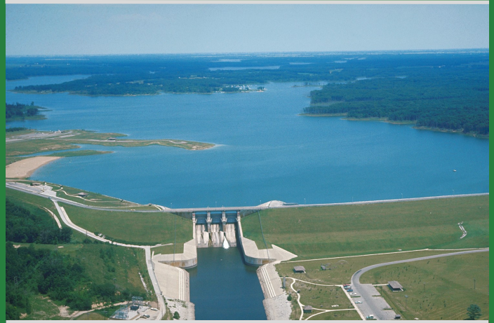
Photo: An aerial image of Lake Shelbyville dam.
